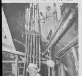
Boilermakers Basilio Maduro (left), and Cleanoutman Thomas Thijzen
